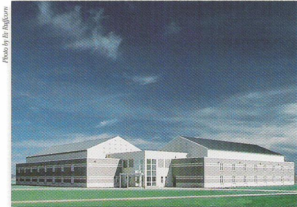
One of the six medium security housing units using CMU for the interior and exterior walls. Concrete masonry lends itself to construction of the most secure buildings without compromising aesthetics.
