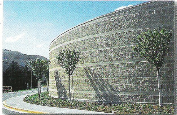
Concrete masonry is used extensively throughout this regional justice center. Curved CMU walls illustrate masonry's design flexibility.
