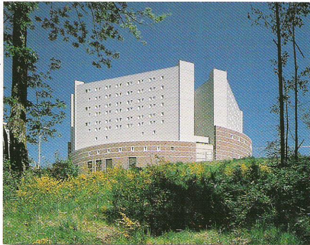
The architectural design of the concrete masonry cylindrical base makes this justice facility's exterior visually attractive. The project received a Construction Specifications Institute award.
