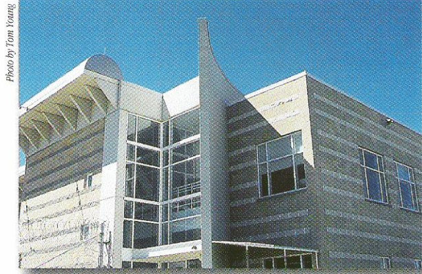
The administration building incorporates an interesting CMU curved wall design which extends from the building's exterior into the interior space. The project's exterior walls were constructed of Hi-R® pre-insulated concrete block for optimum energy efficiency.
