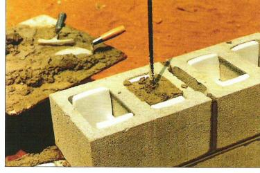
Often relying on the properties of polystyrene, in-core plastic insulation blocks are frequently competitive with insulating concrete forms (ICFs) and structural insulating panels (SIPs) in terms of price. Further, esthetic possibilities are wide-ranging, since there are the same finishes as traditional masonry.
