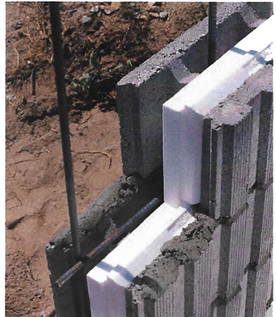
Hi-R masonry wall system with vertical and horizontal steel in place
